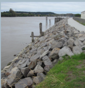
Erosion and flood protection along the northern bank.
